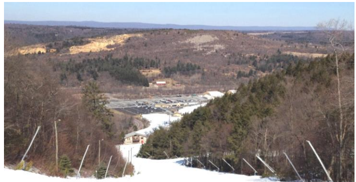
Tight snow gun spacing maximizes production and distribution; located on both sides as appropriate for trail width and wind conditions.
